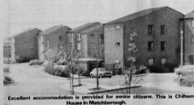
Excellent accommodation is provided for senior citizens. This is Chiltern House in Matchborough.
