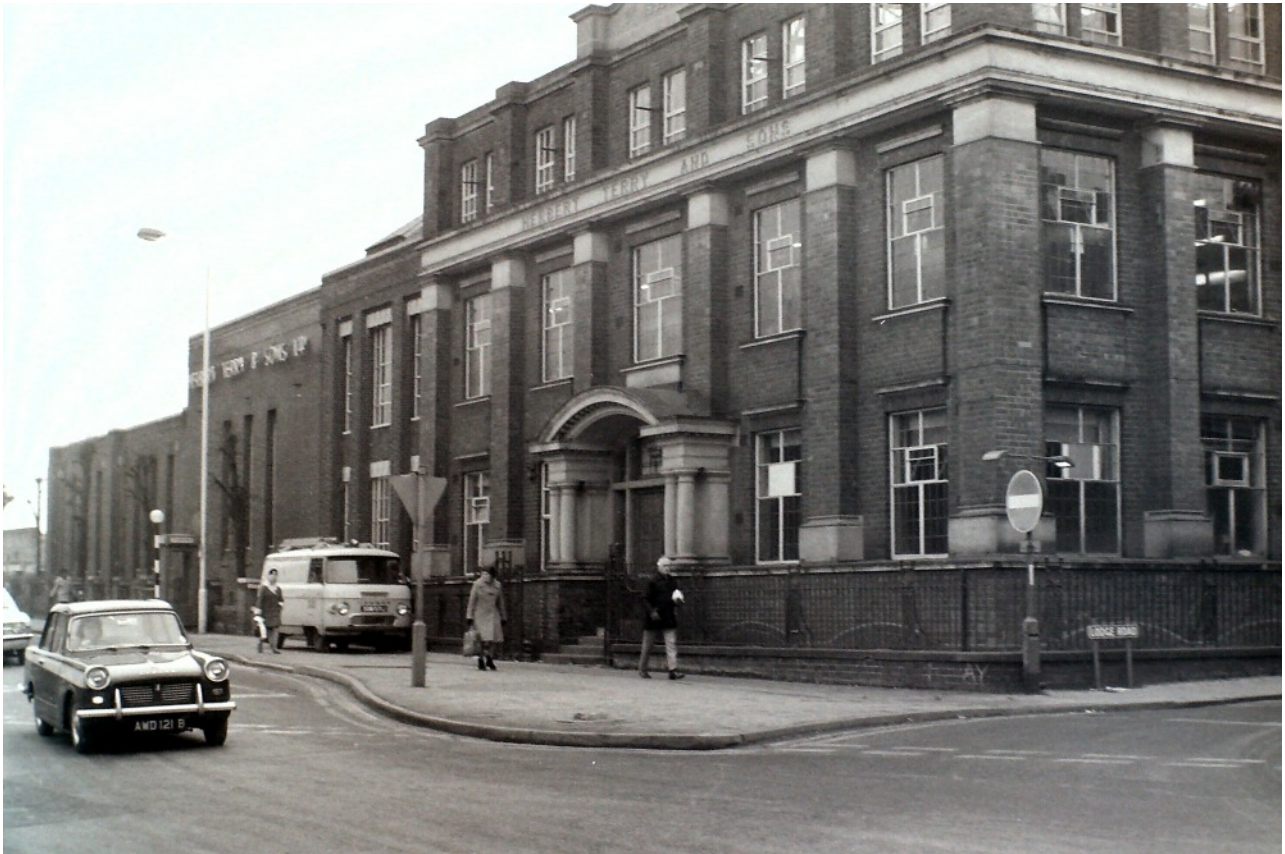
Ipsley Street - Millsborough House looking East.
