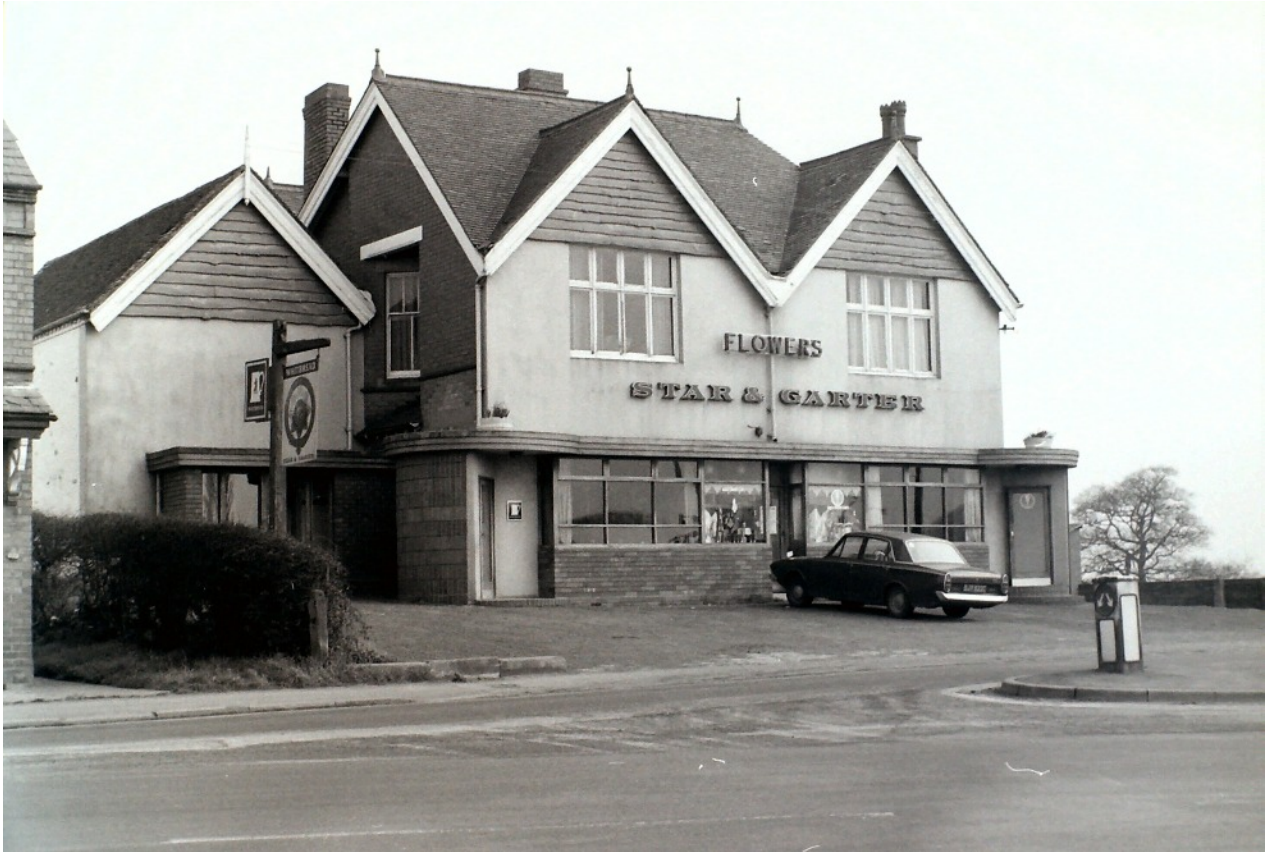
Evesham Road - The Star & Garter Public house.
