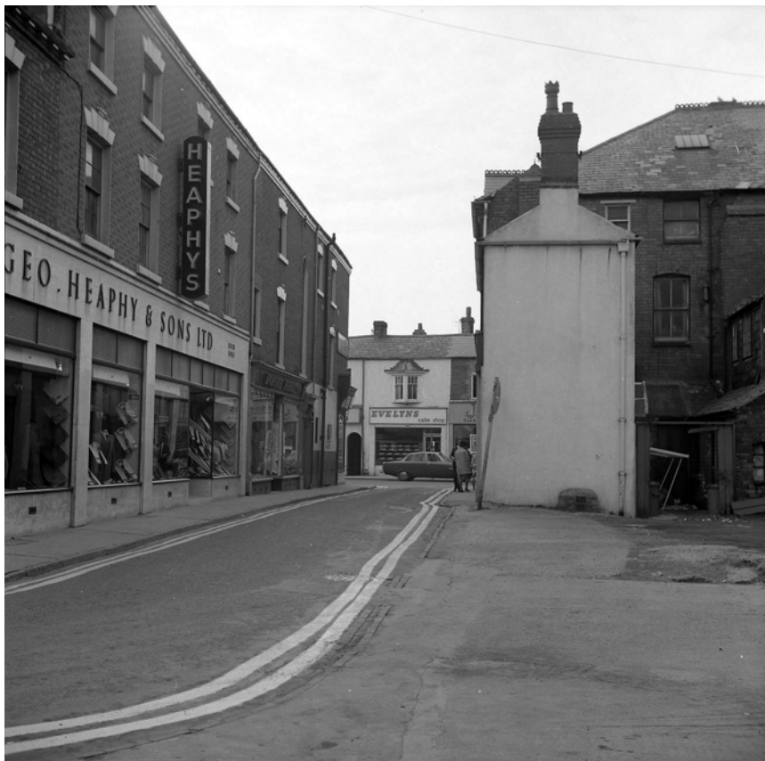
New Street - View from the north side of New Street showing Heaphies Shop and Evehsam Street in the distance.
