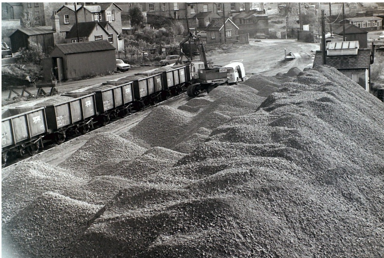
Railway Station - Ballast for building stocked up at the Railway station.
