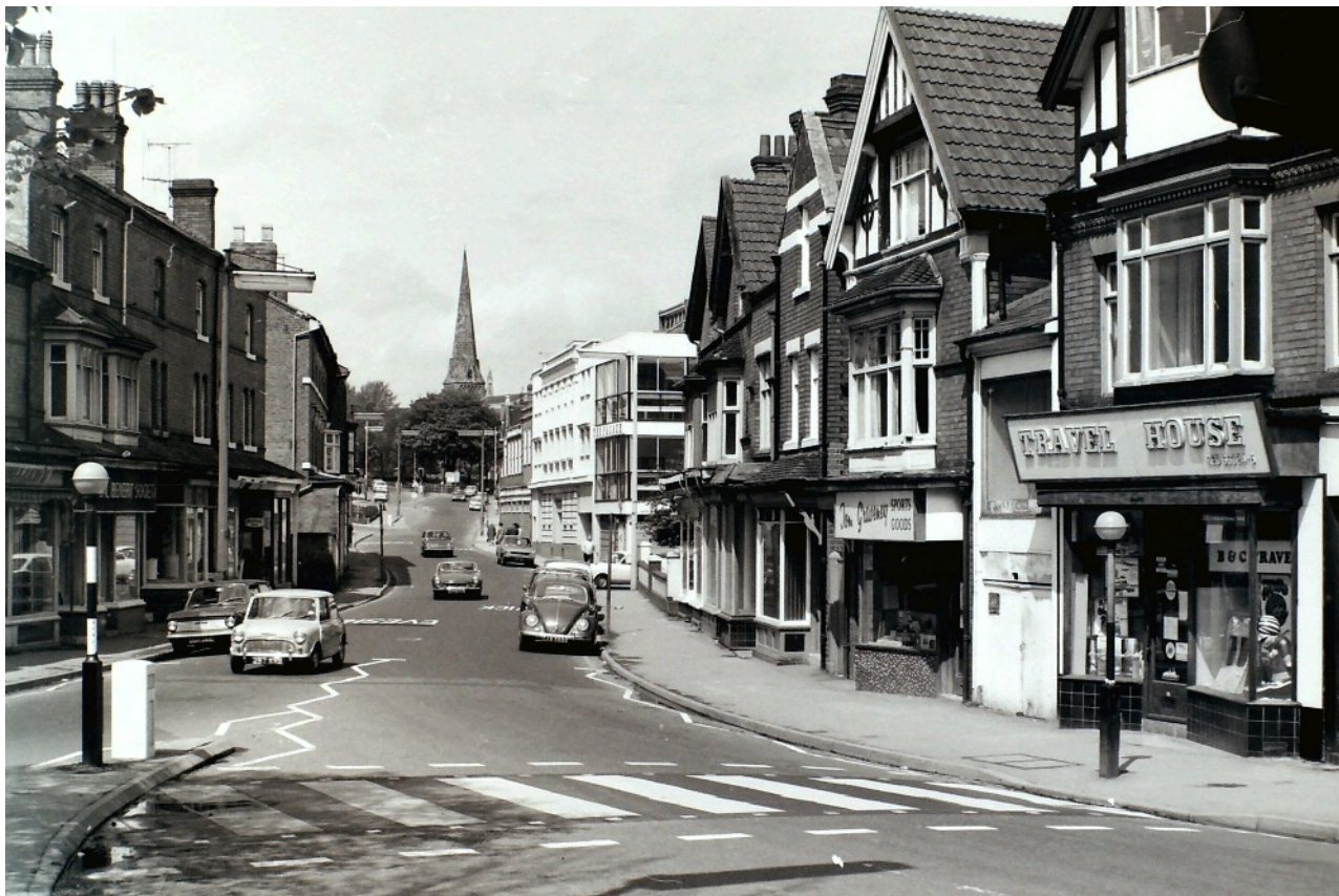
Alcester Street - Looking North on Poole Place up Alcester Street.
